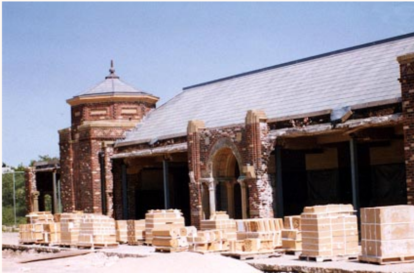
Above is a photo of a well-managed inventory control of many intricate designs. Note the variety of stone, and the positions on the building. This was an historic preservation and reconstruction project. Great care was taken to match all of the original artwork and stone emblems.
