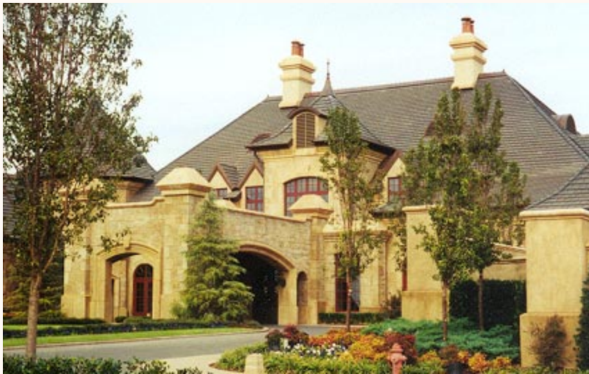
Design stone for the building. Steel reinforcements are usually only needed for balconies and large clear span areas, like the dramatic porte cochere at left.
