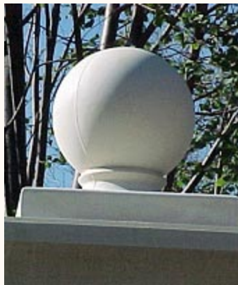
Plastic cast: fast to place. With visible compromises.
