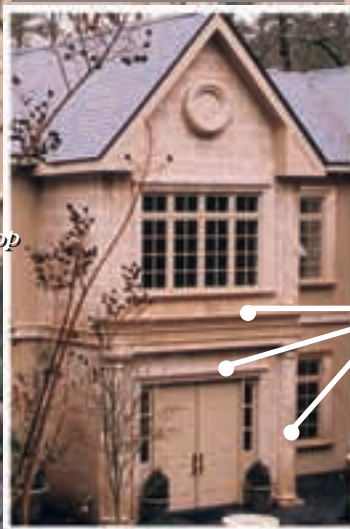
EntryFullFacadeSquare- Top ColumnPilaster EntablatureOrnament Pillared Gable UnitID 131
