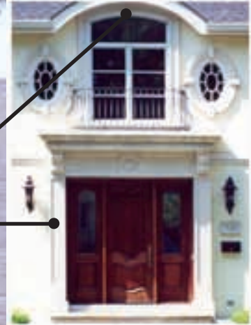
SurroundWindowEyebrow Sill Recess6 Bolson9 UnitID 14052
