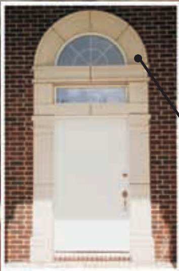
Entry CircleTop ColumnPilaster Justin Crown UnitID 32
